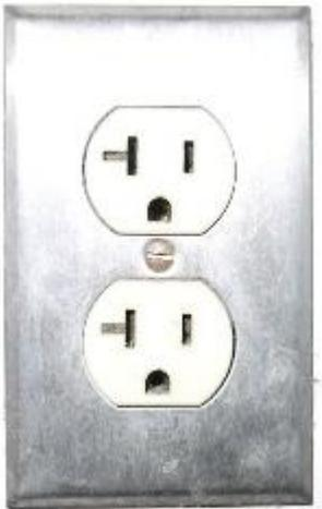
Notice the horizontal notch on the leftmost blade. So instead of being able to draw a de-rated 12A, this plug would enable you to draw a de-rated 16A. You actually get more than the 33% charge increase you'd think you would get since the car uses some power for the computer, so you actually get a 43% boost in charging capacity with this plug. Instead of a most likely 3 miles/hour charge, you'd get 4 or 5 miles/hour.
