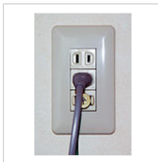
Japanese socket with grounding post, for a washing machine
