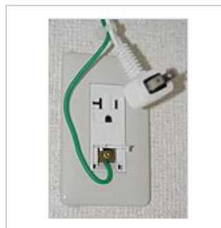
Japanese socket having the narrowest socket face with grounding post, for an air conditioner
