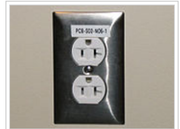
5-20R T-slot receptacle mounted with the ground hole up. The neutral connection is the wider T-shaped slot on the lower right. This is typical for commercial and institutional buildings, outlets in residential buildings are usually oriented differently from this example, so that the ground/earth slot is usually at the bottom.
